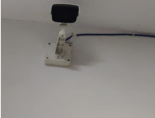
CLOSE CIRCUIT CAMERA
